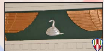
An example of the historic architecture preserved for the Soldiers of the 369th Sustainment Brigade during renovations include columns adorned with rattlesnakes or the regimental distinctive unit insignia, linking back to the 369th Infantry of WWI. The all-black regiment was known as the “Black Rattlers” in 1917.
