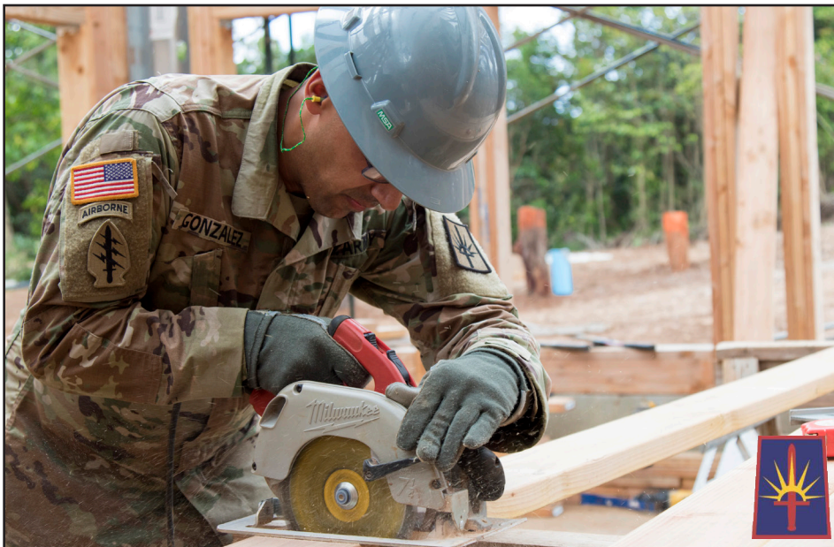
Sgt. Ronald Gonzalez, a wheeled vehicle mechanic assigned to the 1156th Engineer Company, 204th Engineer Battalion, uses a circular saw to cut a board that will be used for framing during Innovative Readiness Training at Girl Scout Camp Paumalu in Haleiwa, Hawaii, July 31, 2019.
