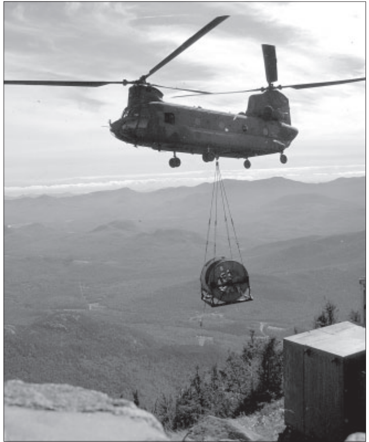
Reaching the 4,867 foot summit, a CH-47 from NY Army Aviation Support Facility #2 lifts a spool of power cable towards Whiteface mountain overlook. Although the winds at the summit measured 25 knots, the aircrew set the cable down with no problems. (Photo by Staff Sgt. Mike R. Smith)
