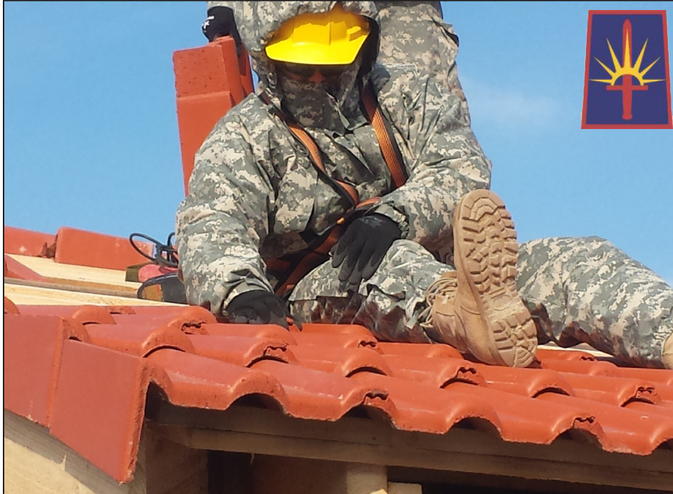
Pfc. Dillon Smith, 1156th Engineer Company, installs European roofing tiles on a building at the Joint Multinational Readiness Center, Hohenfels, Germany, in March. Along with other accomplishments, company troops and two New York Air National Guardsmen constructed two multi-use buildings, complete with wiring during a three-week period. Photo by Capt. Dan Colomb, 1156th Engineer Company.
