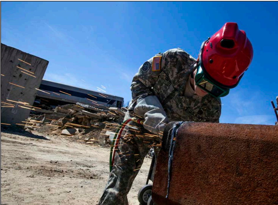
Sgt. Kyle Ortel, Company A, 27th Brigade Special Troops Battalion, New York Army National Guard, cuts a steel pipe with a petrogen torch during a full scale Homeland Response Force exercise involving units from the New Jersey and New York Army and Air National Guard at Joint Base McGuire-Dix-Lakehurst, N.J., April 16. Photo by Master Sgt. Mark C. Olsen.
