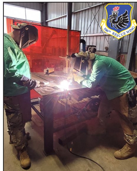
106th Rescue Wing structural specialist engineers practice welding at the Silver Flag exercise at Tyndall Air Force Base, Panama City, Florida, Jan. 10, 2022. Courtesy photo.
