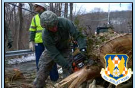
An Airmen from the 105th Airlift Wing clears debris from a road in the town of Carmel, N.Y. on March 5.
